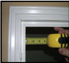
Measure Right & Top frame for spacing.
