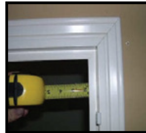
Measure Left & Top frame for spacing.
