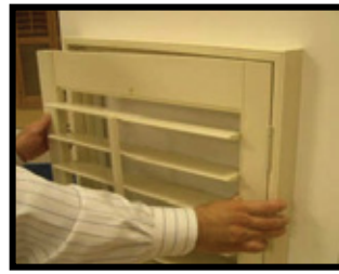
Insert hinge side panel into position first.
