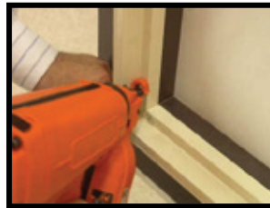
Only secure one nail or screw into the Bottom left frame.
