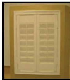
Slide panel into frame hinges and close other panel to hold in place.
