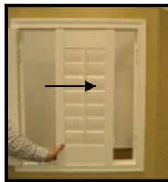
Position panel in the frame.
